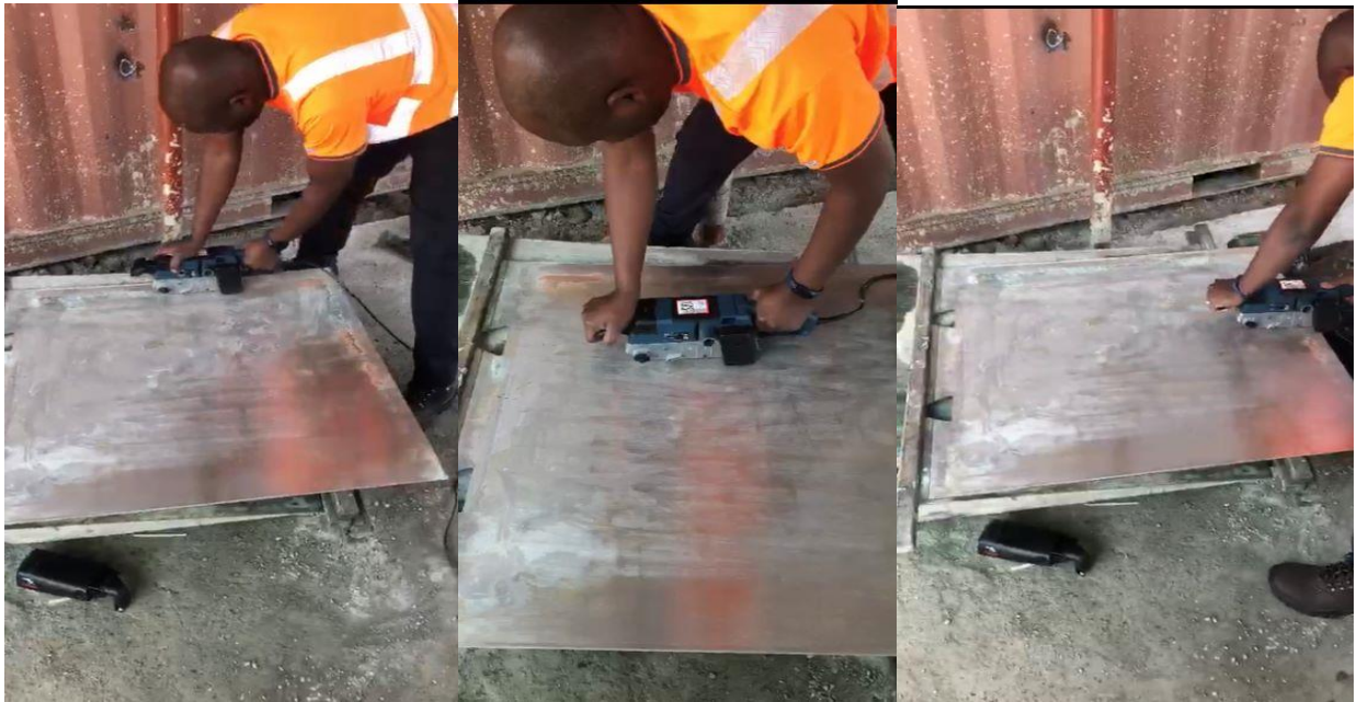
Edge Strip Removal and Surface Preparation
